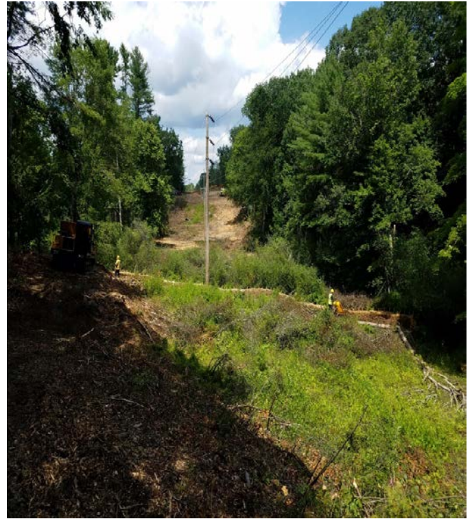
Fig 22: BMP installation south of Oyster River. Viewing north. (7-24-19).
