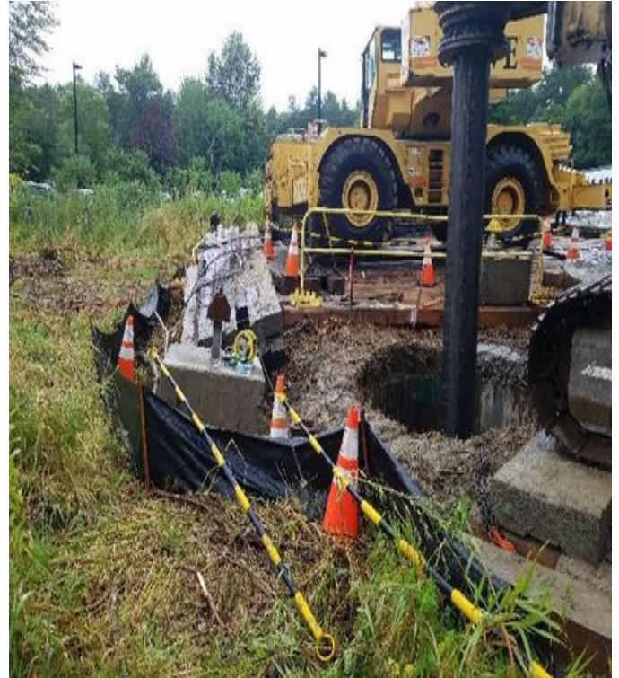
Fig 18: MJ is drilling Str. 23, next to wetland DW67. Viewing west. (7-23-19).
