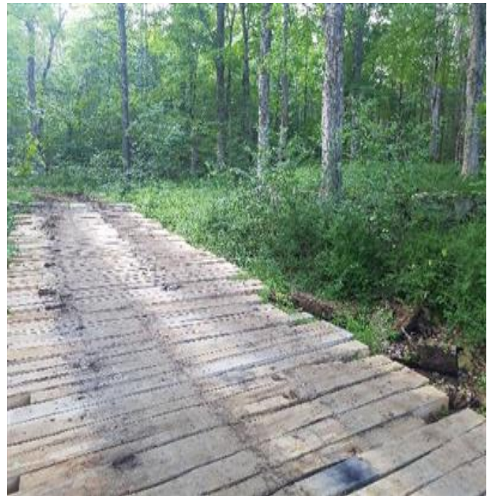
Fig 6: Foss Farm access road, near graveyard. Viewing east. (7-19-19).
