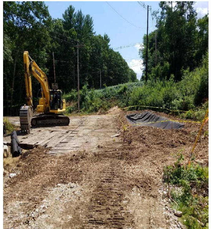
Fig 24: Dewatering basin at Str. 32. Viewing south. (7-24-19).
