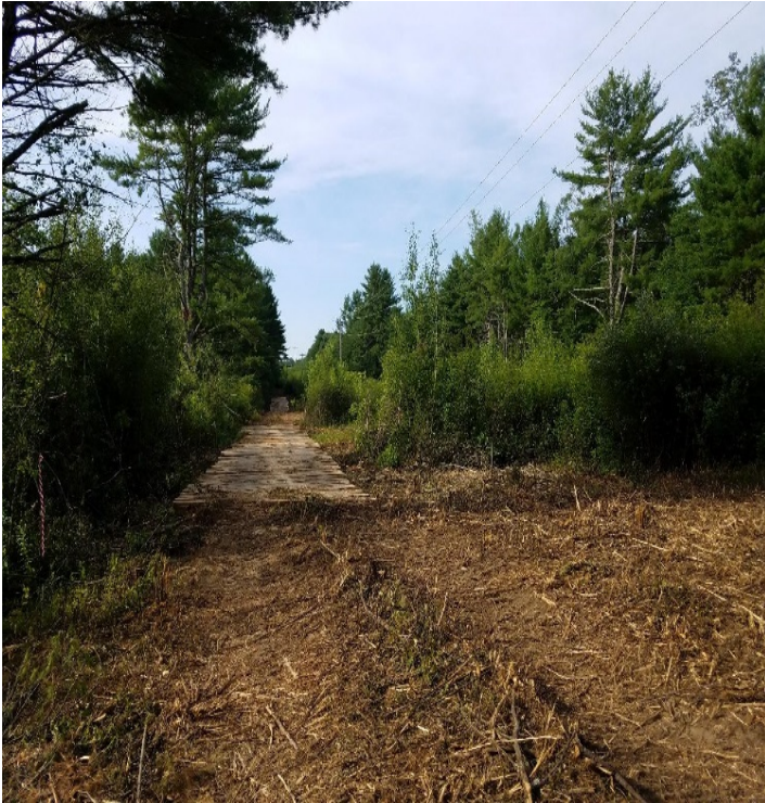
Fig 13: Timber matting over northern portion of wetland DW58. Viewing south (7-22-19).
