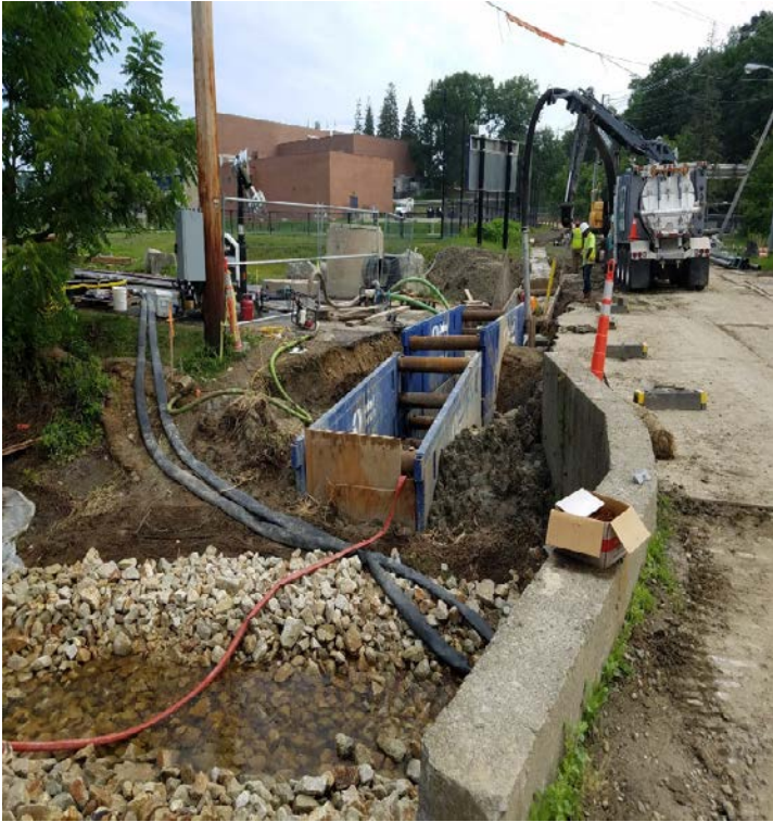
Fig 21: Pouring float fill in trench, north of College Brook. Viewing north. (7-24-19).
