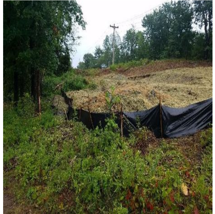
Fig 20: Silt fence on the downslope area where soils are being Spread near Str. 27. Viewing north. (7-23-19).
