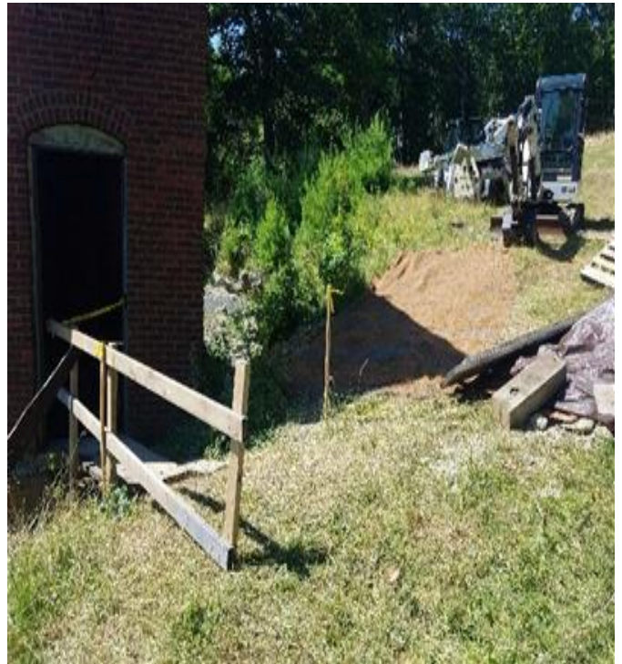
Fig 8: Gratan removing debris from around the cable house. Viewing south. (7-19-19).
