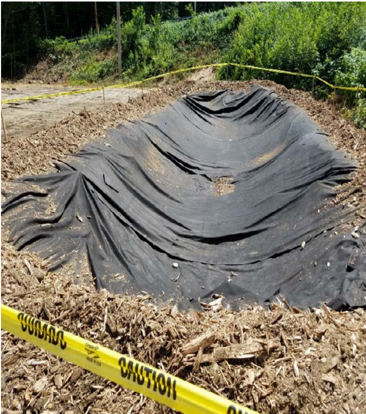
Fig 25: 25'X50'X4' dewatering basin, lined with filter fabric. Viewing south. (7-24-19).
