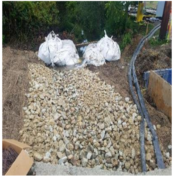
Fig 2: Temporary filter fabric and stone installed in College brook. Viewing west. (7-18-19).
