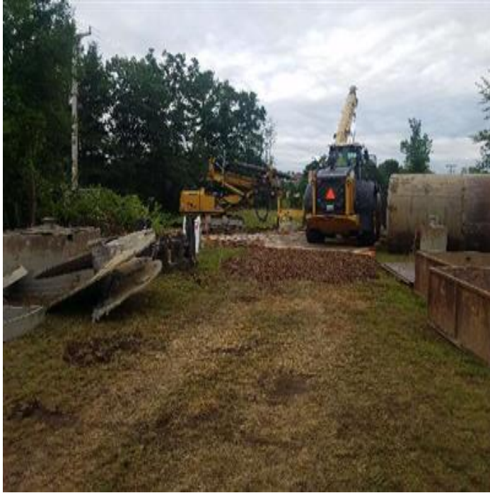
Fig 1: MJ staging equipment, prepping to drill Str. 23. Viewing south. (7-18-19).
