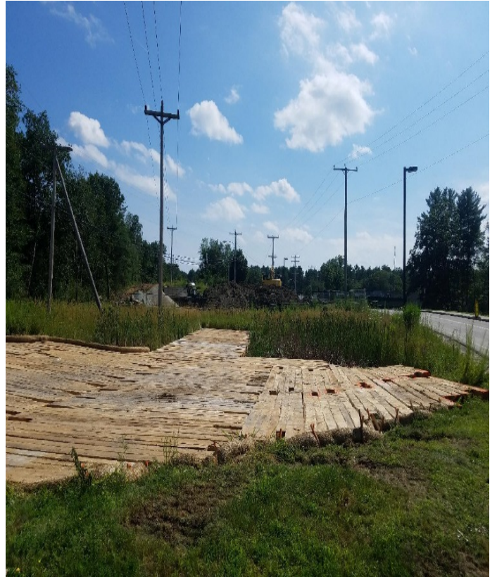
Fig 4: Str. 24 work pad within wetland DW65. Viewing south. (7-19-19).
