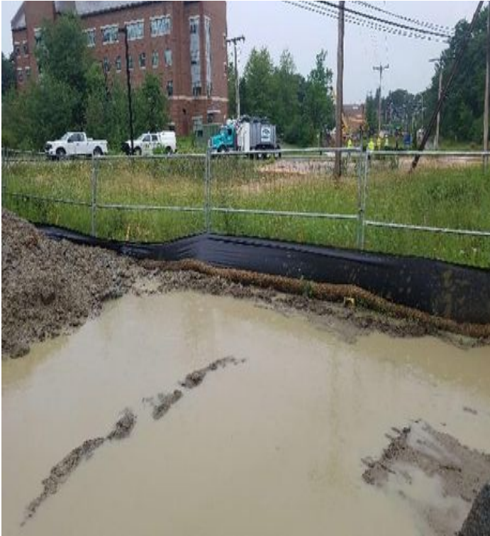
Fig 17: Low area in Waterworks Rd laydown yard that requires straw bales. Viewing north. (7-23-19).
