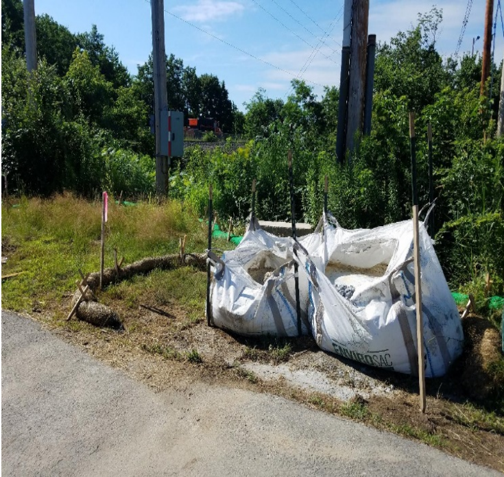
Fig 5: Concrete wash out station with perimeter BMPs installed. Viewing southeast. (7-19-19)
